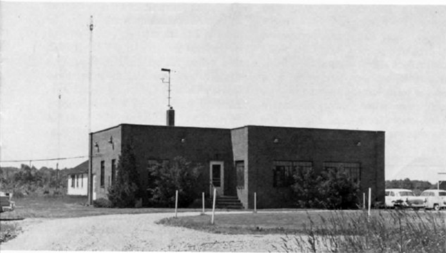
■ Located two miles west of Lorain, Ohio, in an open field, this inconspicuous building is a beehive of activity all year round. Even during the slow winter months, staff members are busy servicing equipment to keep it in tip-top shape.
